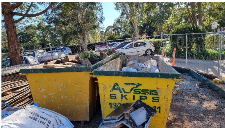
Plate 5. Dedicated and secured waste storage area
