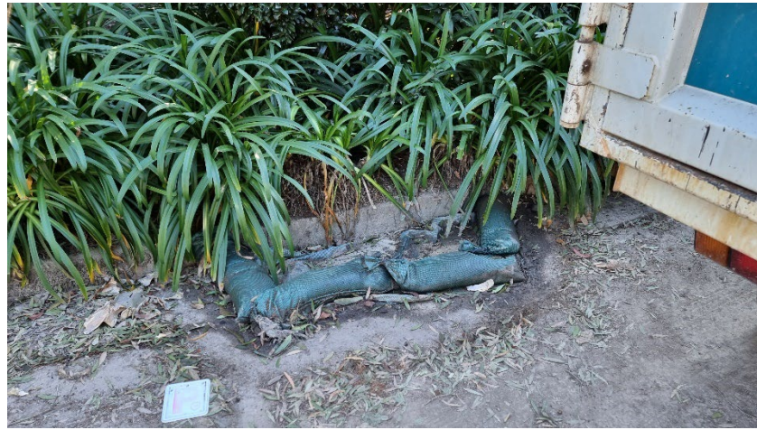
Plate 1. Sediment trap around the stormwater inlet in carpark
