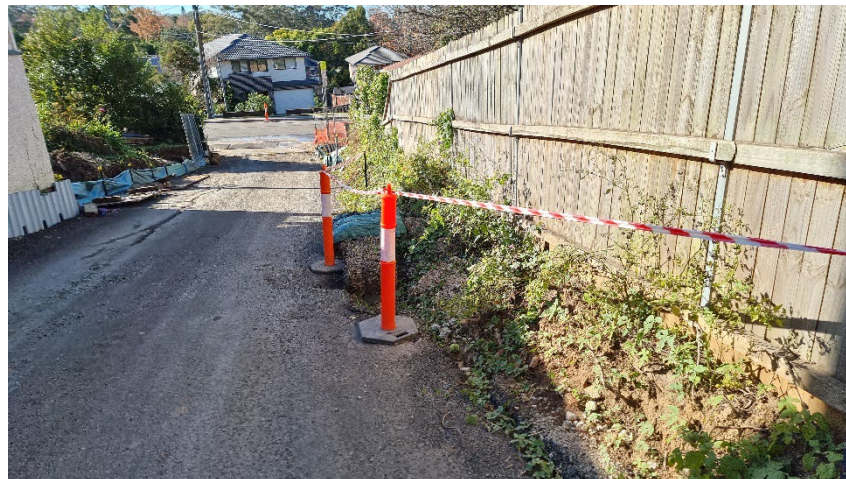
Plate 2. Sediment fencing and check dams on driveway edge
