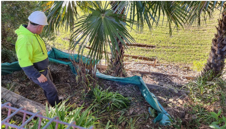
Plate 3. Established surface water point from active work area across vegetated areas
