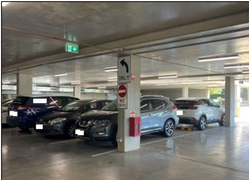
Plate P4. Directional Signage in the new carpark; firefighting equipment/signage
