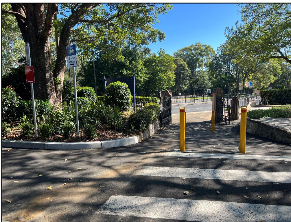
Plate P8. Bollards installed at heritage gate.
