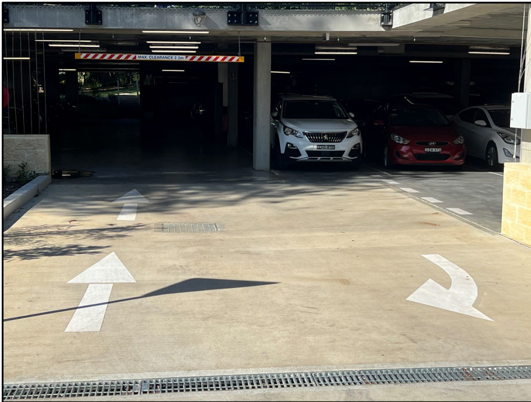
Plate P3. Carpark directional signage for entry /exit
