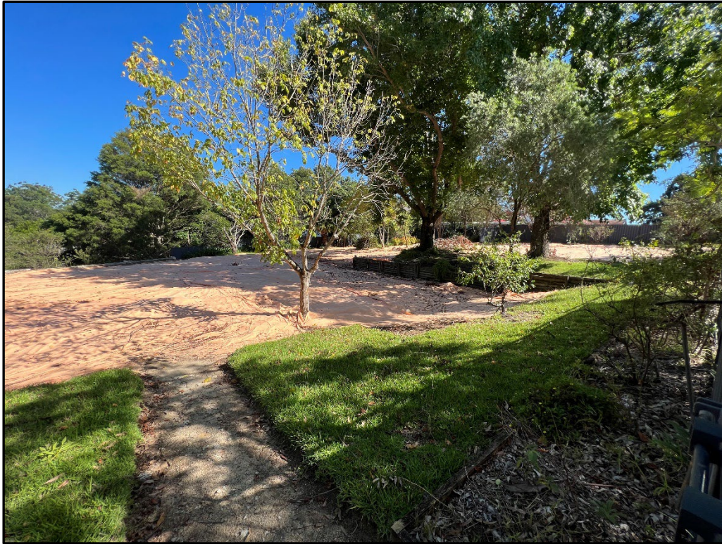
Plate P9. Substage 4 – Geofab installed over exposed soil
